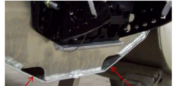
Large drains to remove water
