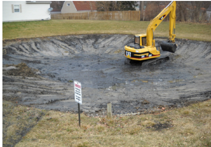
Figure 2. One of the Foxwood Villa stormwater ponds in the midst of a dredge operation (City of Toledo Engineering Service 2015).
