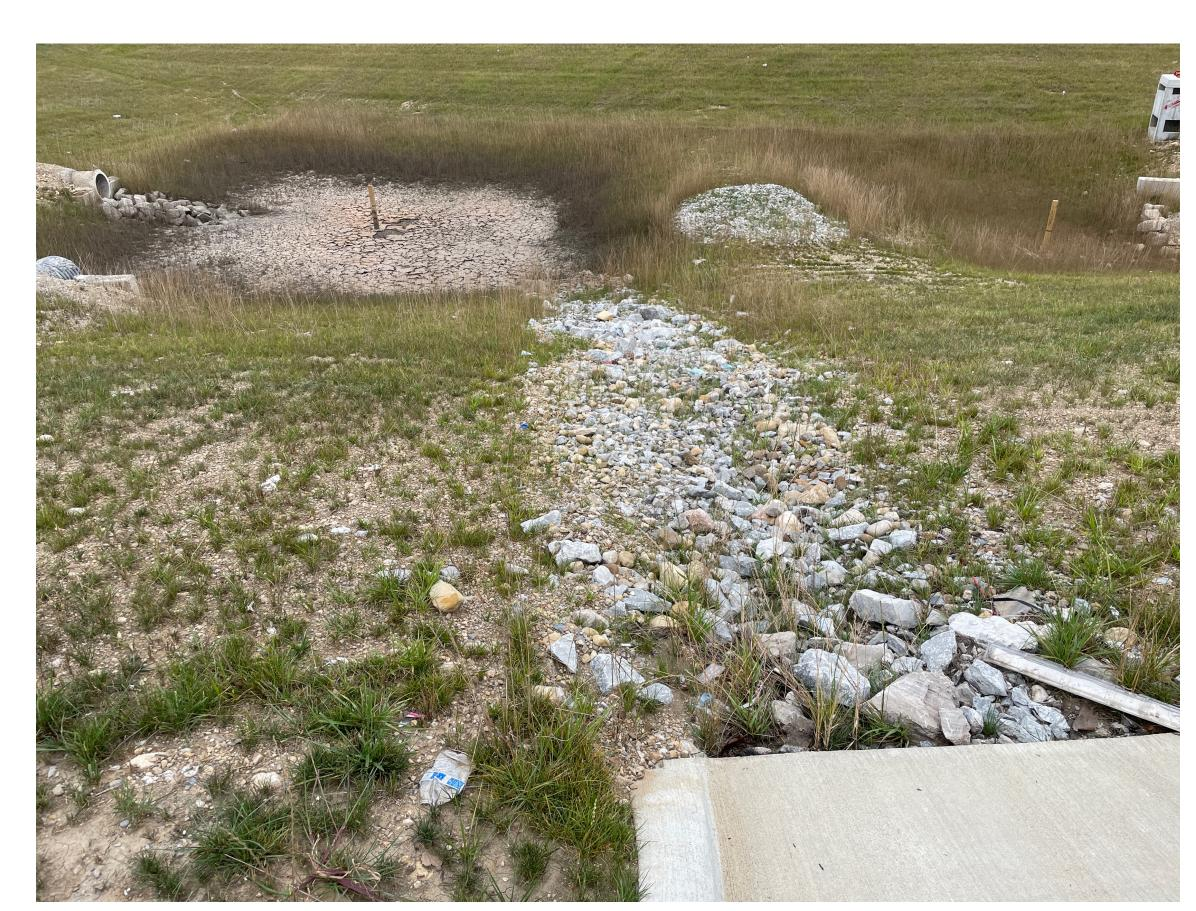
This is a dried-out stormwater catch basin. When it rains, this valley-like area is where most of the water from the facility drains to. When it starts raining, the spouts are where I collect the water for testing.
